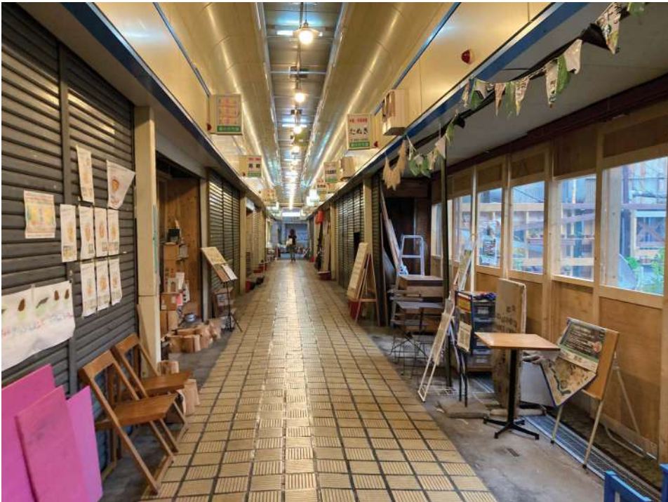
FIGURE 11.6 The Nada Central market in need of reconstruction for disaster preparedness and the entrance of Ichibatake to the right side. (Taken by the author.)
